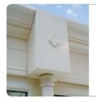
Gutter outlets are fully sealed and can accommodate a full range of decorative aluminium hoppers and downpipes.
