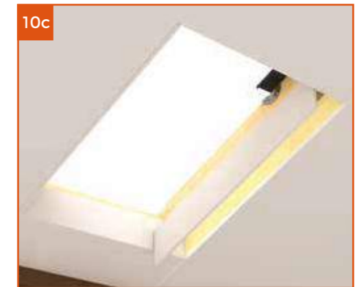
Finish around the roof window opening with plasterboard.
