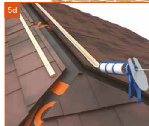
Use low module silicone between the back edge of the roof batten and tile.
