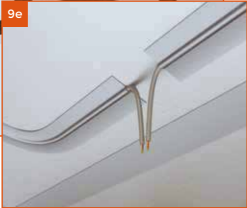
At this point, any wiring for lighting/spotlights should be added.
