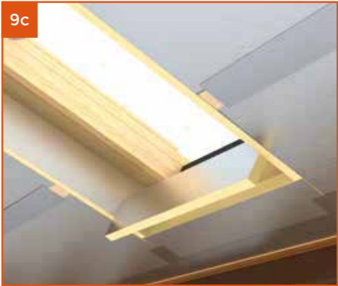
Seal around roof window with 25mm insulation.
