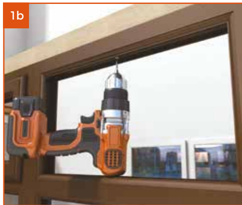
1b Remove existing glazing and fix through timber packer using fixings supplied. Fixings at no more than 150mm from either end and no more than 500mm centres.
