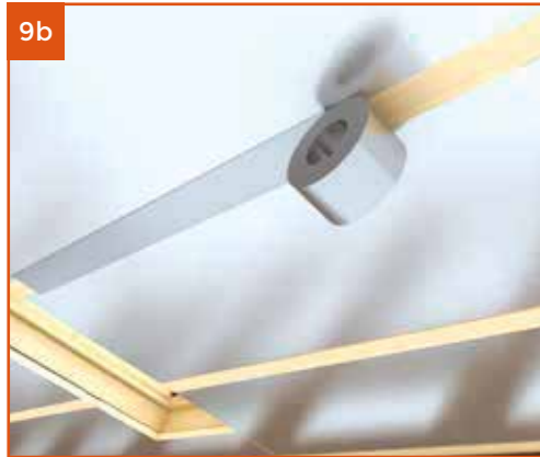
Insulation tape should be run over every batten and the window line so no timber will be visible from the inside.
