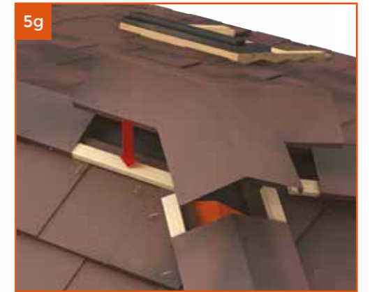
Fix rafter cap over delta ridge profile at verge and fix on all sides. Use touch up kit provided to hide screw heads.
