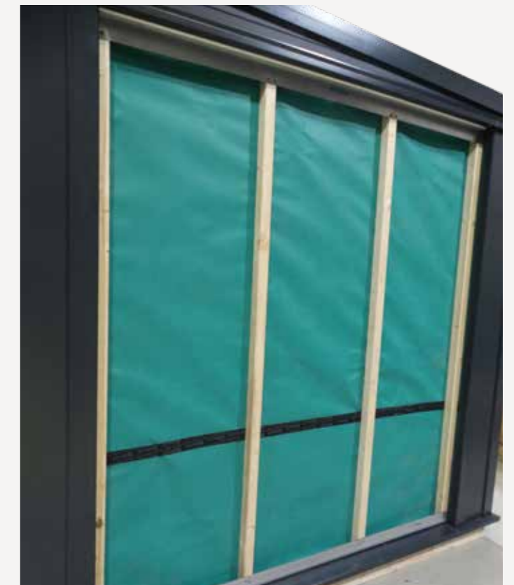
Wall prepared for cladding - battens supplied
