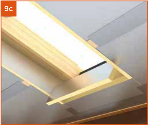
Seal around roof window with 25mm insulation.
