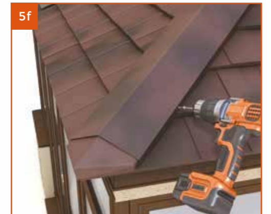
Position delta ridge over batten and fix side on. Use touch up kit provided to hide screw heads.
