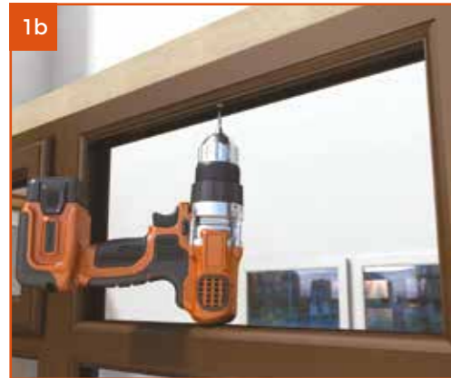
1b Remove existing glazing and fix through timber packer using fixings supplied. Fixings at no more than 150mm from either end and no more than 500mm centres.
