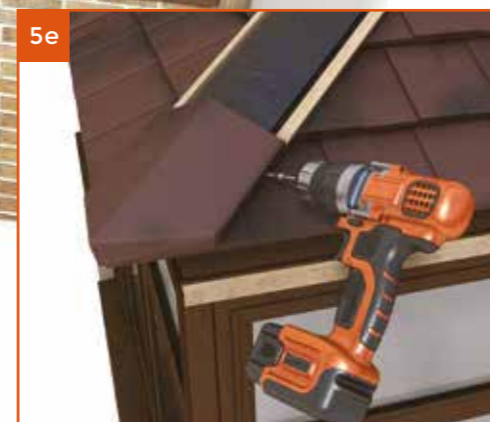
Fit endcaps and fix on both sides. Use touch up kit provided to hide screw heads.
