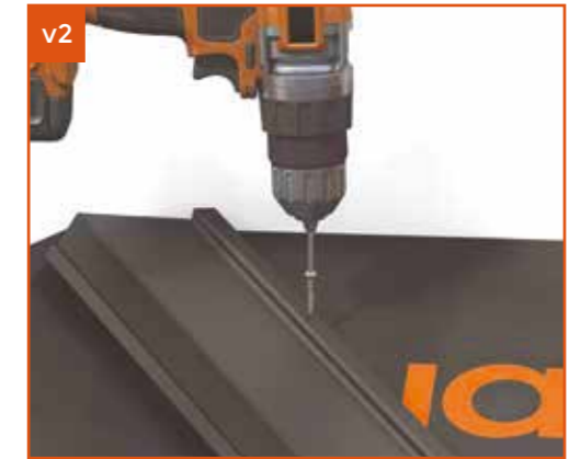
v2 Fix the valley flashing using self-tapping screws.
