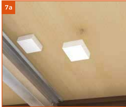
Apply foam packers to the exposed screw heads under the ply, ensuring that the foam packers are evenly spaced.
