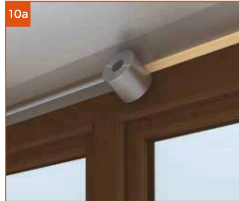
Insulated tape should be used around the top of the window frames to cover any exposed timber.
